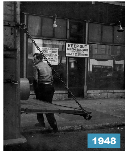
Photos 1-3. Demolition for the Congress Street Expressway
